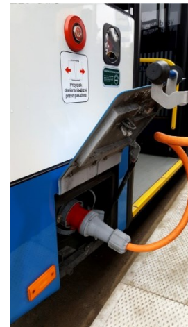
Fig. 7. Charging of traction batteries from 400 VAC grid on a terminus
