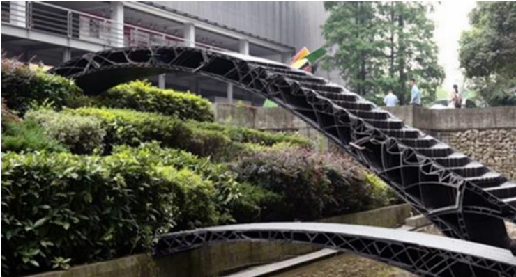
Fig. 13. A pedestrian bridge made of plastic in the 3D print technology, where the span measures 11 meters
