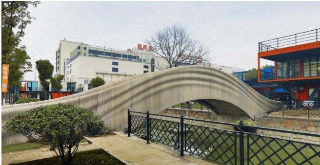
Fig. 10. Shanghai – a concrete bridge with a 26 meters long span is currently the longest bridge made in the 3D print technology.
