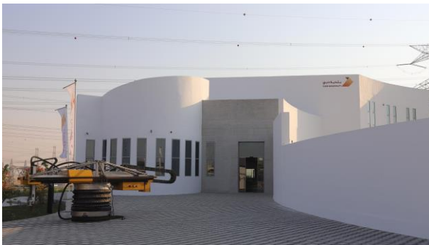
Fig. 6. A facility made in the 3DP technology in Dubai [2]
