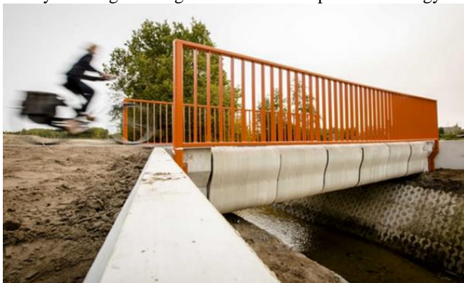
Fig. 11. A prestressed concrete bike bridge in the Netherlands, reinforced with fibers
