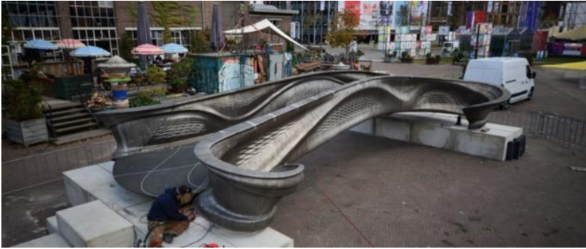
Fig. 12. A stainless-steel bridge construction, made with the use of an automated 3D print technology
