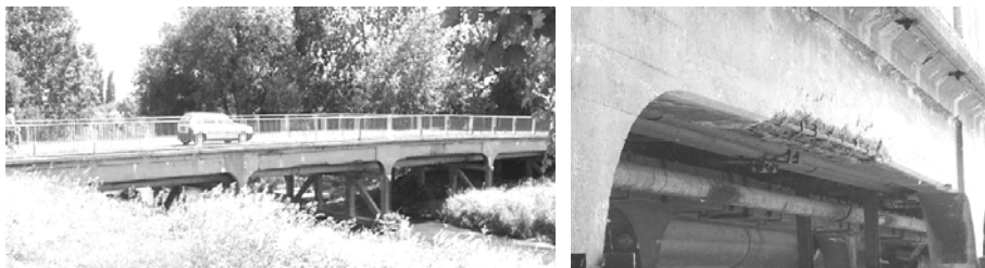
Fig. 9-10. Kalinowszczyzna Bridge, 1908, in-flow views
