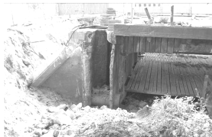
Fig 16. Double wall creates the abutment corps
