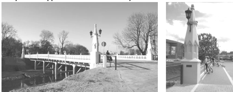
Fig. 19-20. After the refurbishment, April of 2012
