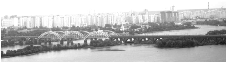
Fig. 5. The present view at the Darnytskyi Bridges, 2012
