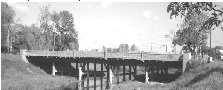
Fig. 11. Old Bridge, at 1909, from inflow view
