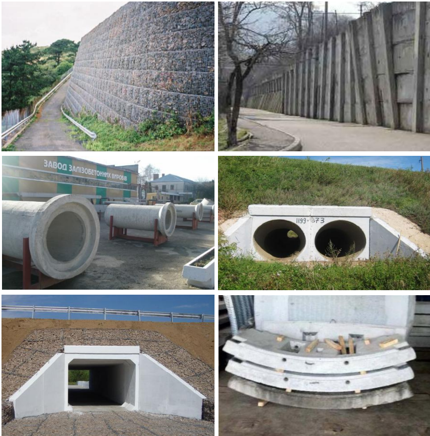
Fig. 1. Road traffic facilities:
