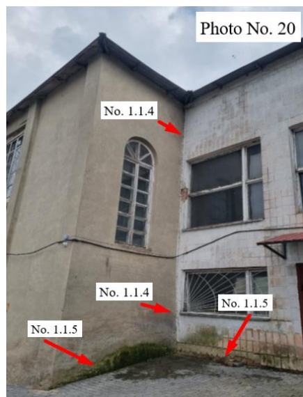
Fig. 1. Cracks ( a , b ) and dampness ( b ) on the outer side of the walls
