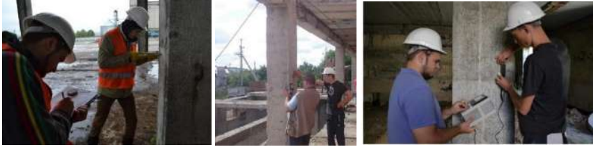
Fig. 6. Instrumental examination of columns
