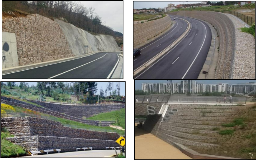
Fig. 1. Examples of gabion retaining walls [6]
