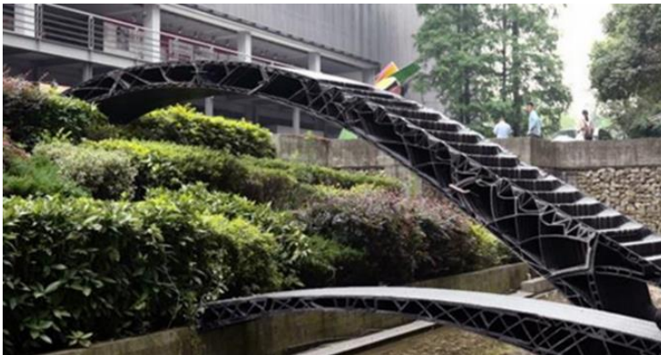
Fig. 13. A pedestrian bridge made of plastic in the 3D print technology, where the span measures 11 meters
