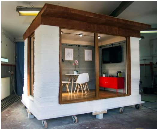
Fig. 8. The first house created in the 3DP technology in Poland
