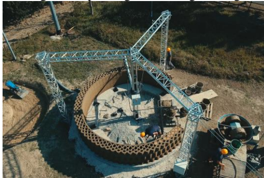
Fig. 5. Construction industry 3DP in-situ
