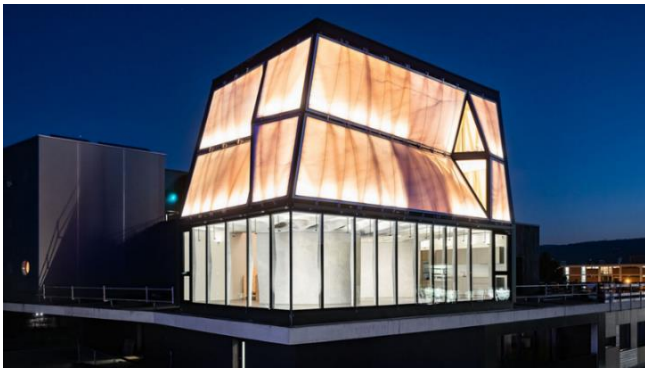
Fig. 9. DFAB House, in Dübendorf – the first inhabited house made in a 3DP technology
